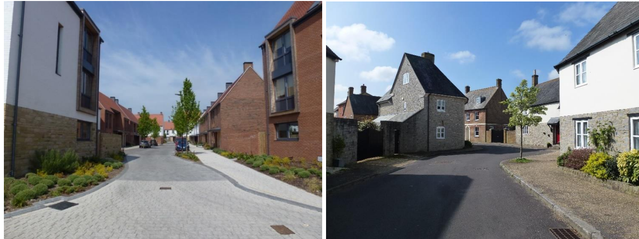
Figure 5-9: Carriageway deflection, sharp corner radii, street trees and changes in material all help reduce speeds in residential streets. L: Poundbury, Dorset. R: Derwenthorpe, York (Credit - Andy Cameron)
