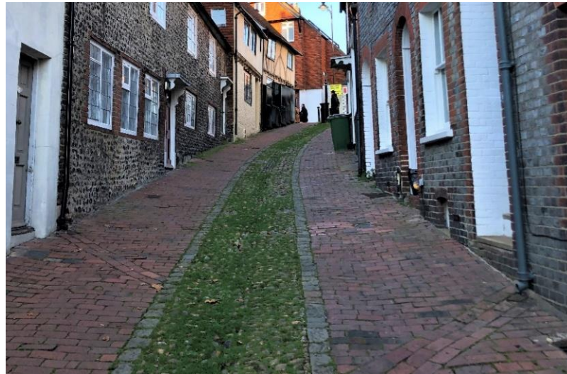
Figure 8-8: Cobble channel in narrow street, Lewes, Sussex. Note the lateral channels directing flows from RWPs. (Credit - Create Streets)
