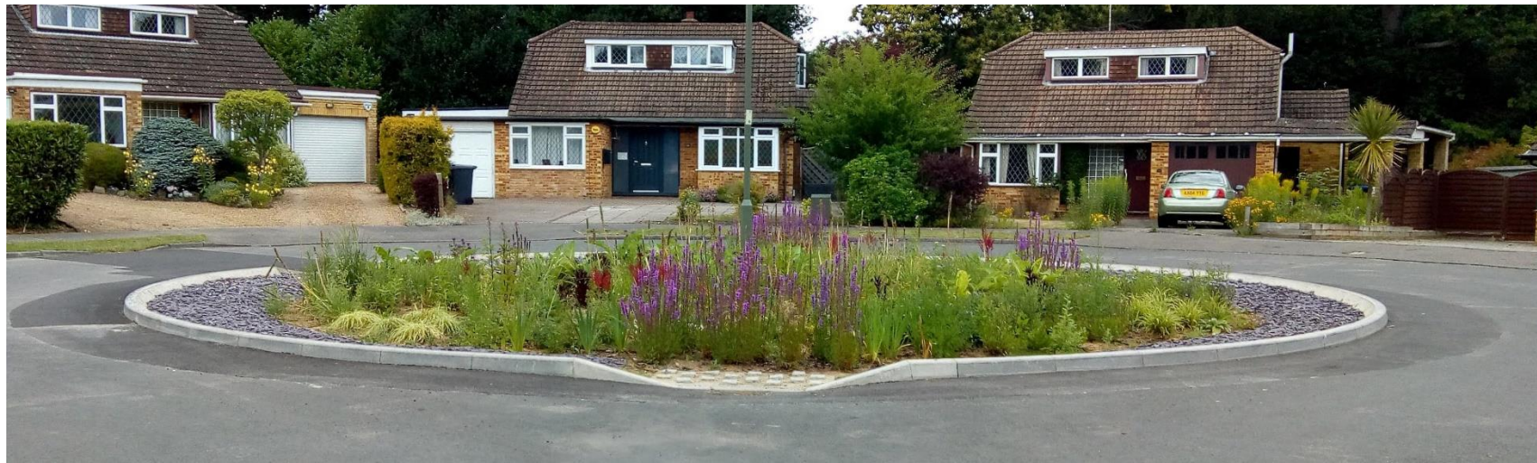
Fig 8-5: Left over areas grass can be re-purposed into rain gardens with wildflowers, Blackdown Close, Woking, Surrey (Credit - SCC)
