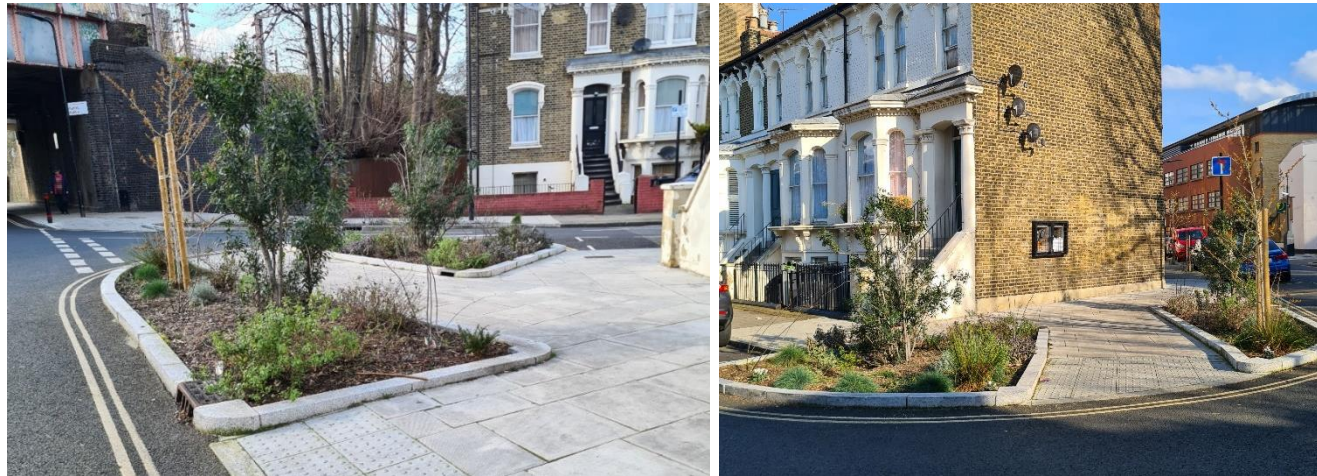
Figure 5-8: Reduced kerb radii improves pedestrian crossing and provides additional space for greening. (Credit - Create Streets)
